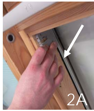
Remove any existing brackets from the window frame.
