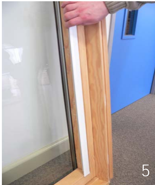
Place R/H side channel against window frame.
