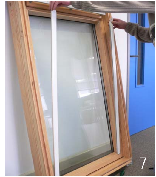
Gently pull the side channels away from the top of the window frame.
